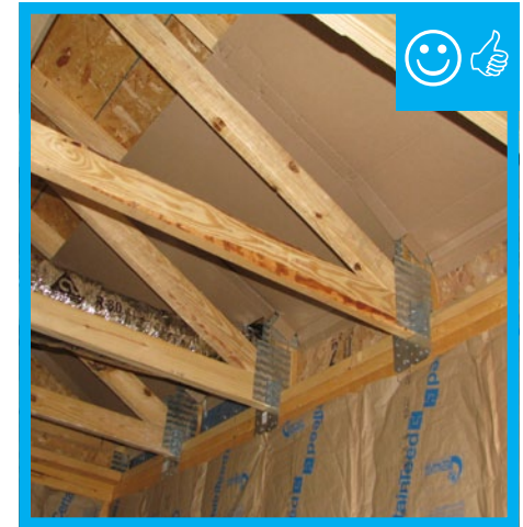
Framing and wind baffle installation will allow for required insulation depth.
