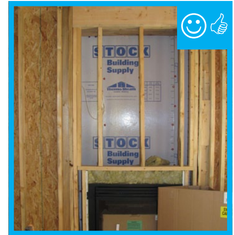
Rigid air barrier is installed behind fireplace.
