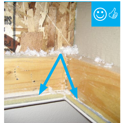
From inside attic: this attic access door has a foam and rubber weather-stripping installed that remains in contact when closed.
