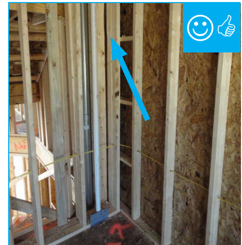
Gap in framing will allow for corner to be filled with insulation.
