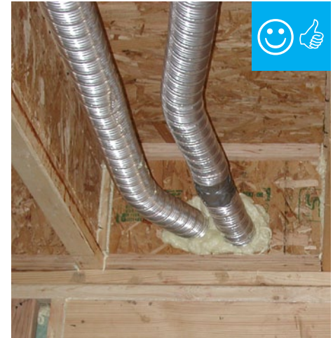
Neatly cut and sealed penetration.
