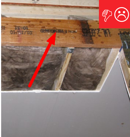
A. No gasket installed at marriage wall connection prior to assembly.
