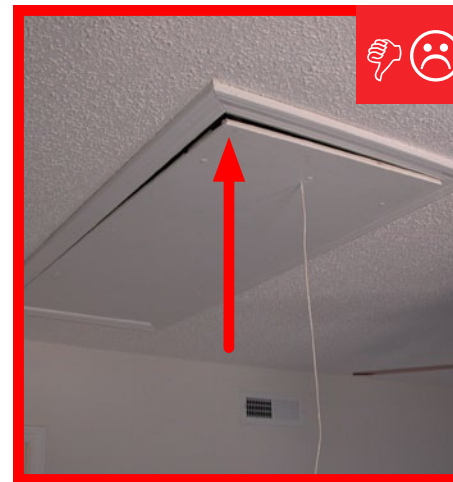
C./D. There is no weather stripping or gasket around the attic stair hatch.
