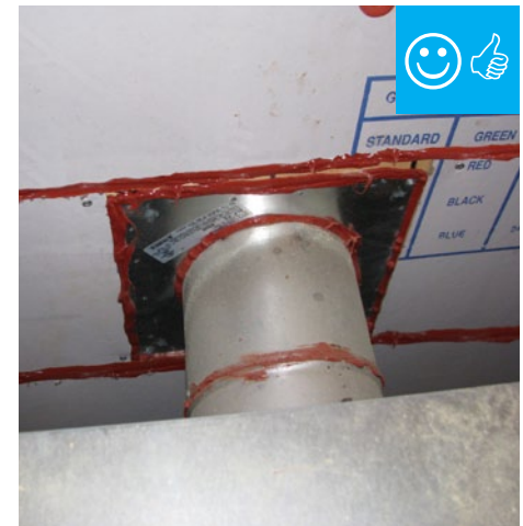
Vent and air barrier sealed.
