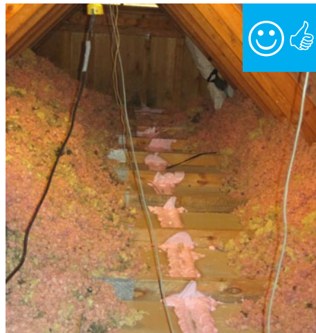
Top plate to drywall connection sealed from attic with foam sealant.
