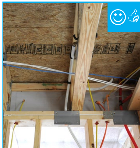
Air barrier and penetrations sealed between porch attic and conditioned space.
