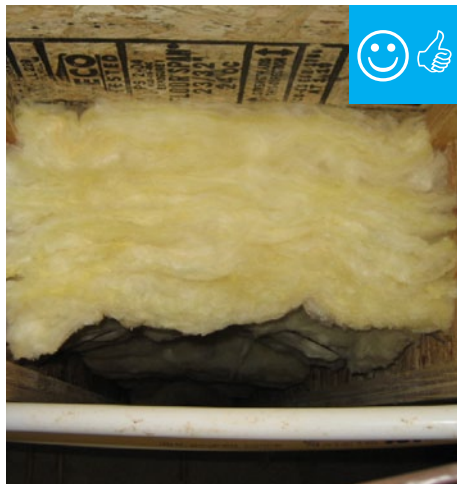
Sub-floor insulation is properly installed and supported.
