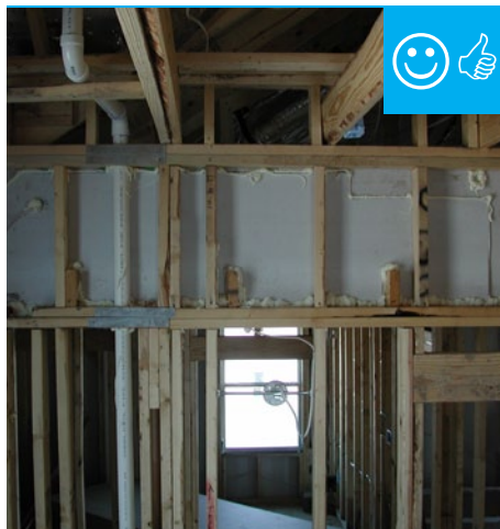
Backing air sealed prior to insulation.
