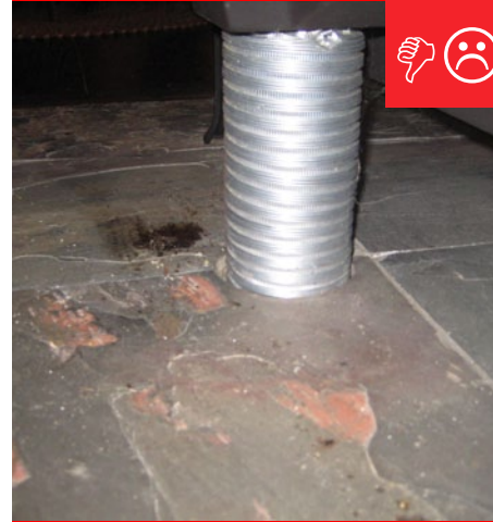
B. Penetration through the floor is not air sealed.
