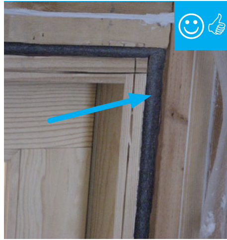
Rough opening around window has been filled with backer-rod to air seal.
