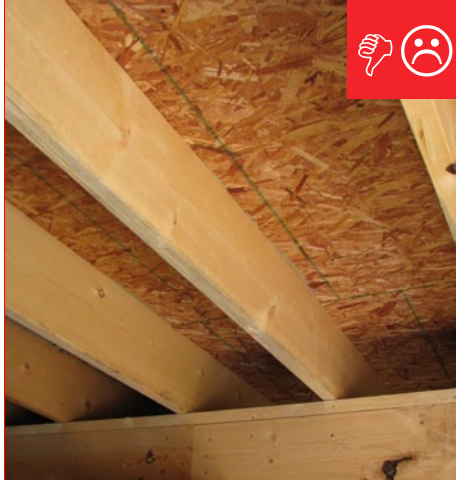
A. No air barrier is present between the floor system and unconditioned space.
