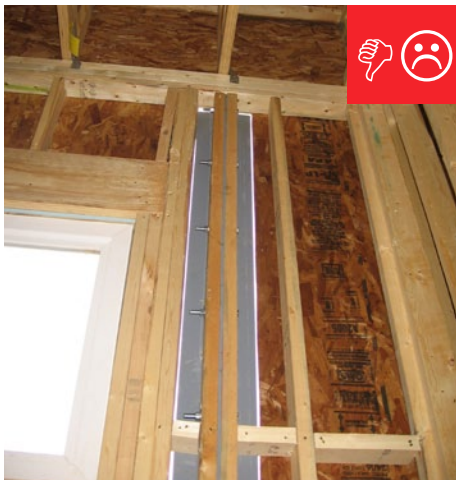
B. Air barrier is air sealed.
