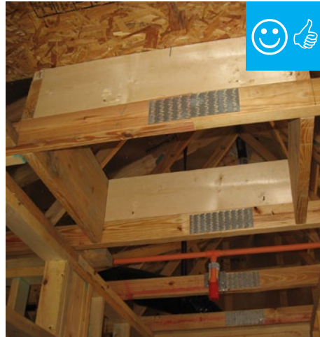
Blocking has been installed around the perimeter of this attic access to prevent insulation falling into the house.
