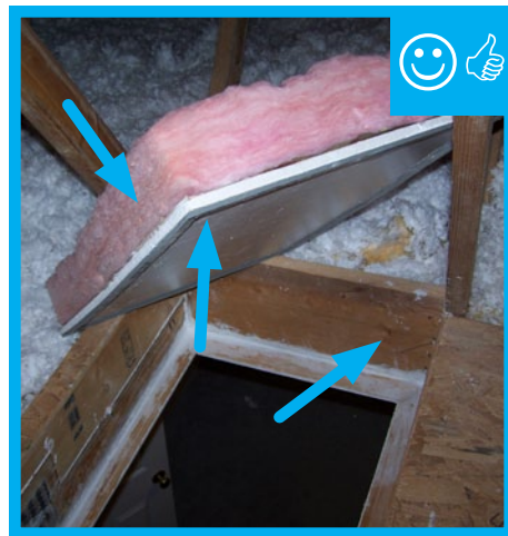
Attic access hatch has been properly insulated by attaching a fiberglass batt, gasketed, and opening has blocking.
