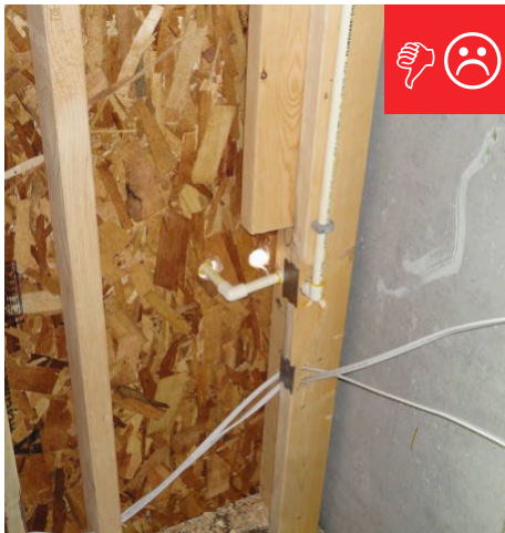
B. Framing does not allow for corner to be insulated.
