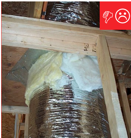
C. Fibrous insulation does not air seal.
