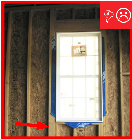
A. Window has an additional non-structural king stud.
