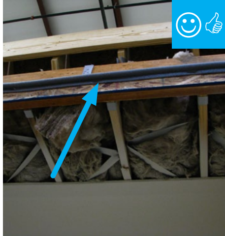
Gasket installed at marriage wall connection prior to assembling modules.
