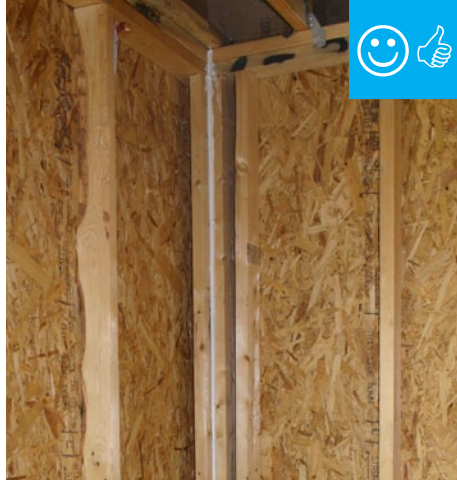
Framing allows for corner to be insulated.
