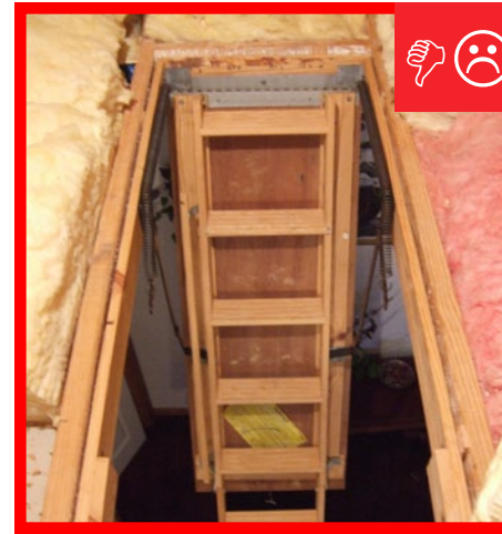
B. Drop down stairs do not have an insulation cover installed.
