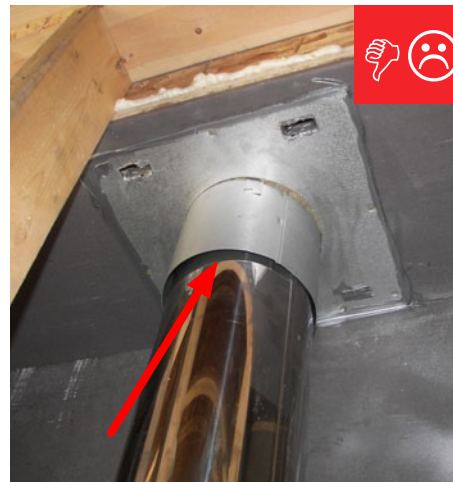
D. Vent sleeve not completely sealed.
