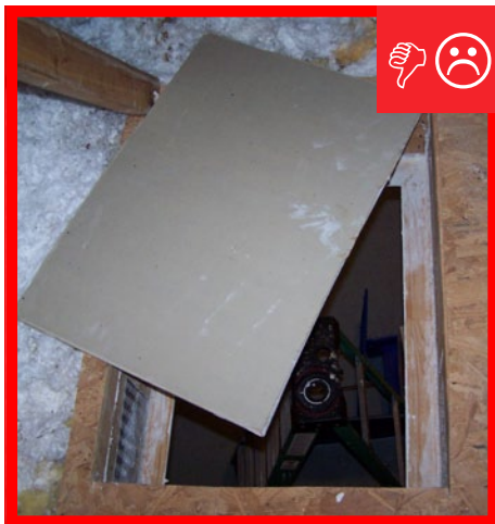
B. Attic access panel does not have an insulation cover installed.
