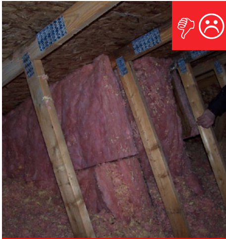
A. Rigid air barrier not installed to hold insulation in place.
