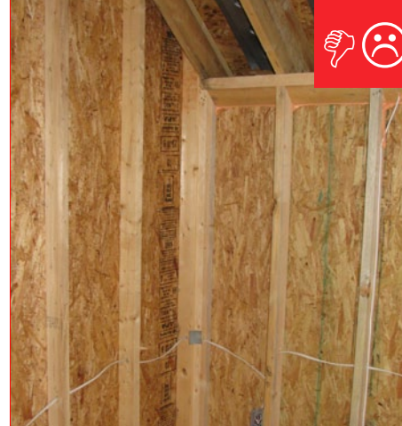
A. Framing does not allow for corner to be insulated.
