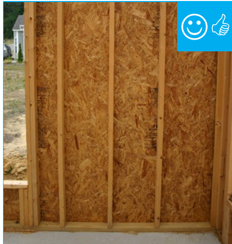
Continuous air barrier
