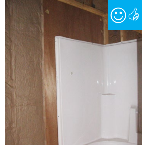
Air barrier installed behind shower stall.
