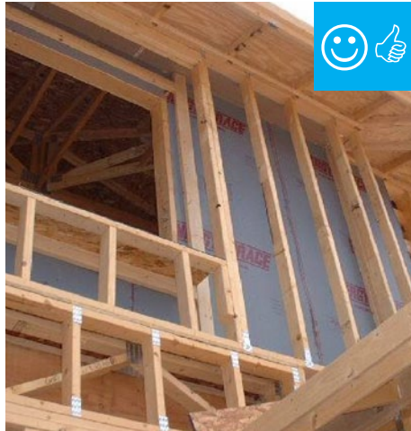
Air barrier is installed between double-wall framing.
