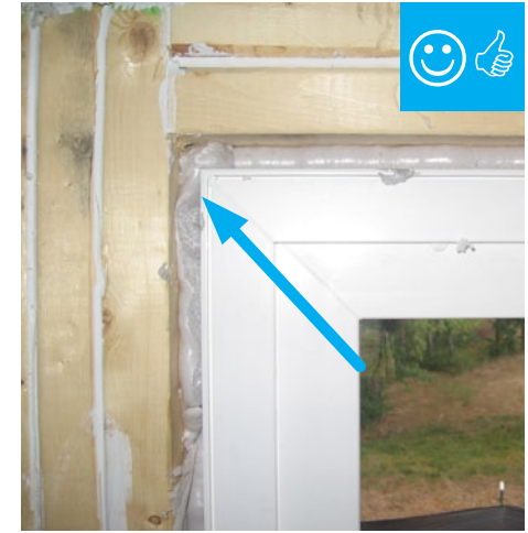
Rough opening around window has been filled with low-expansion foam to air seal.
