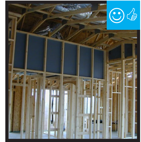
Rigid backing installed prior to insulation.
