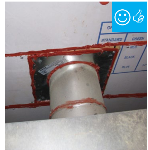
Vent and air barrier sealed.
