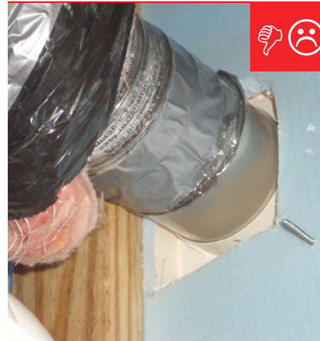
B. Penetration hole is larger than duct and not sealed.
