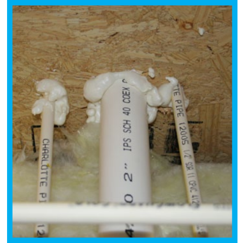
Penetrations through floor are air sealed.
