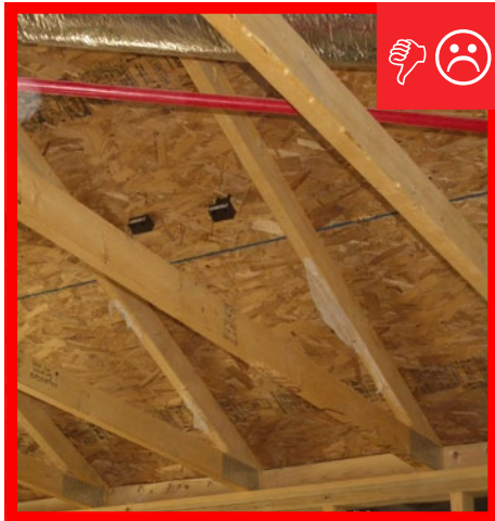
A. Framing will not allow for required insulation depth.
