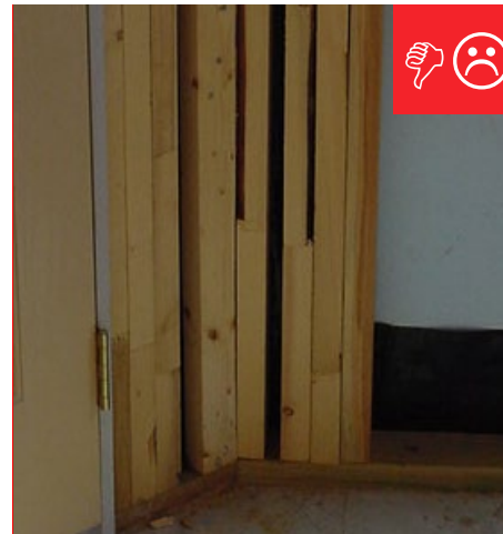
B. Excessive framing will not allow for corner to be insulated.
