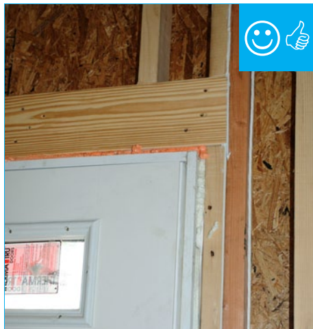
Appropriate door framing installed.
