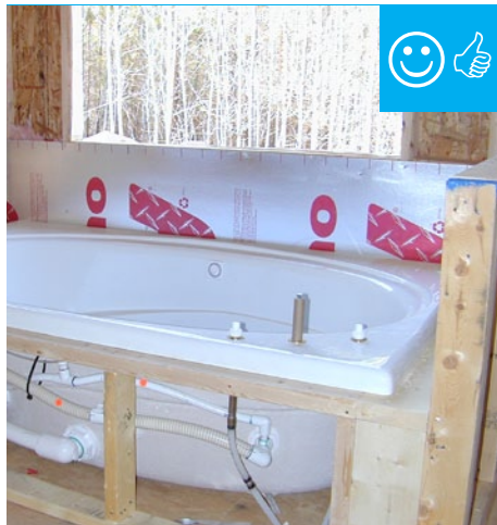
Air barrier installed behind the tub.
