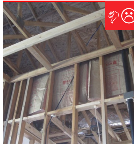
B. No rigid backing on knee wall.
