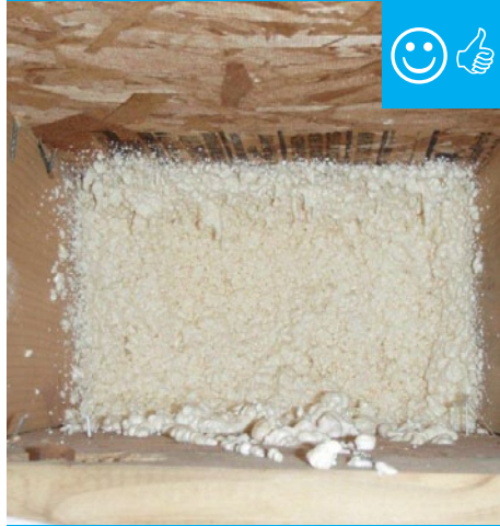
Air barrier is present and installed between the floor system and unconditioned space.
