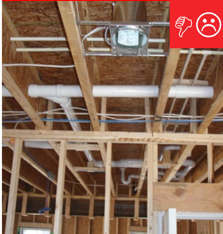
A. Floor system does not have air barrier to separate it from garage.
