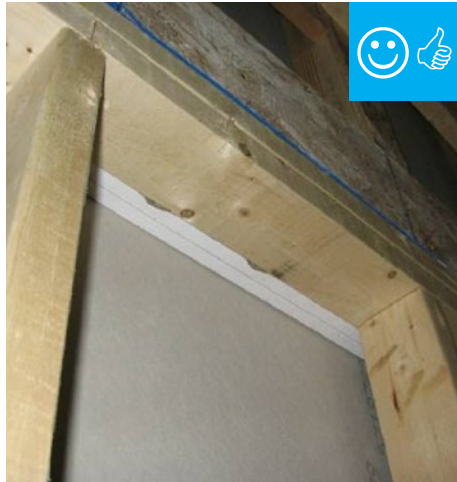
Approved common assembly installed.
