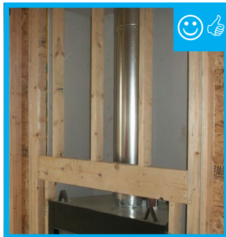
Rigid air barrier is installed behind fireplace.
