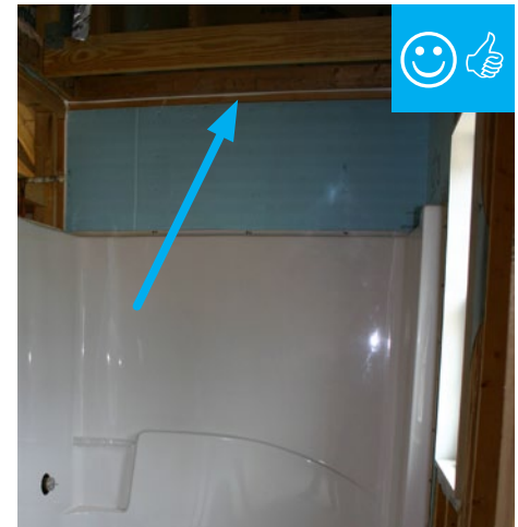
Air barrier sealed.
