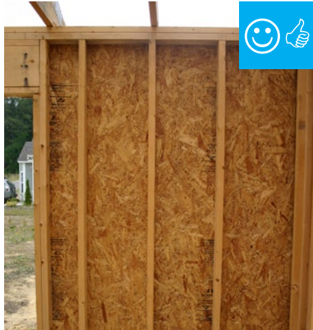
Proper spacing of 2 x 4 studs.
