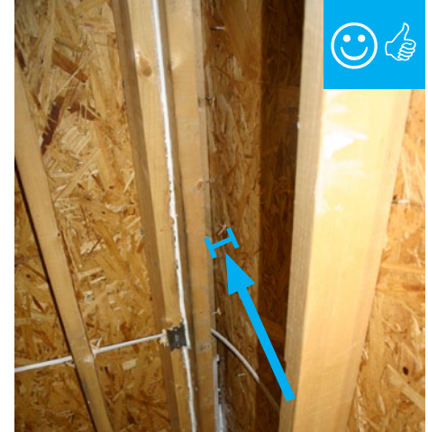
Framing does allows for corner to be insulated.
