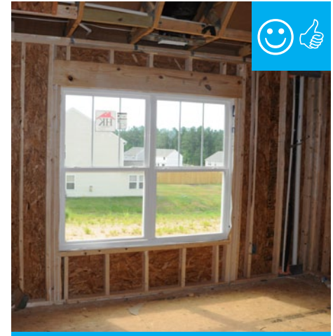
Appropriate use of framing members to support double windows and additional cripples for drywall purposes.
