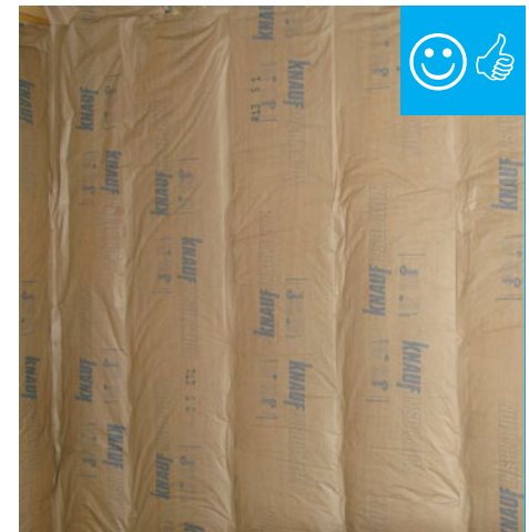
Insulation is properly installed.
