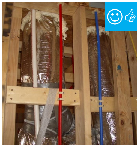
Penetrations have been neatly cut and properly sealed with foam.
