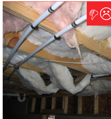
D. Sub-floor insulation is not properly installed or supported.
