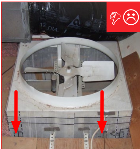
C. Whole house fan installed with holes in surrounding platform that need to be air sealed.
