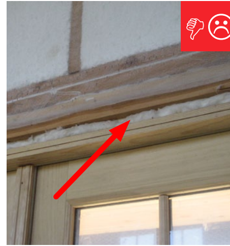
B. Fibrous insulation is not an air barrier and cannot be used to air seal openings.
