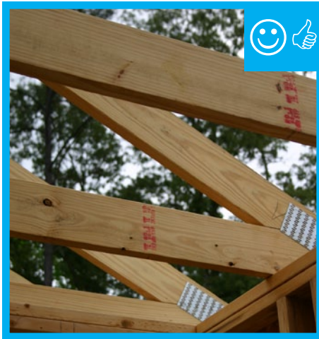
Framing allows for required insulation depth.
