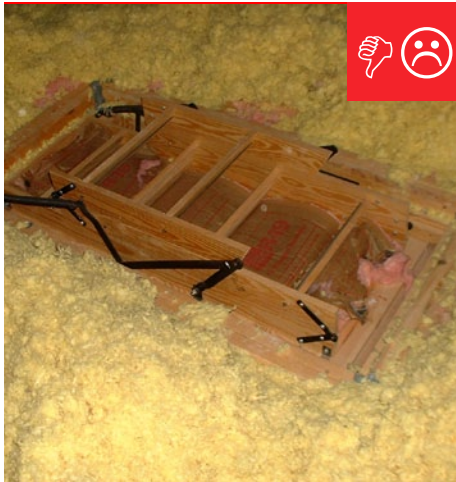
A. No blocking installed to prevent attic insulation from falling into stairs and opening.
